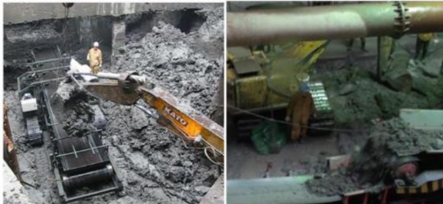
Figure 7. Field tests of the track-type belt conveyor.
